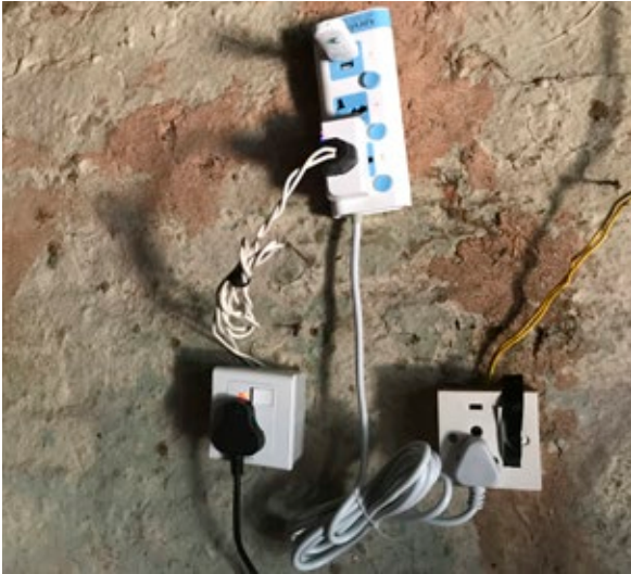
Power meter connected to an induction stove
