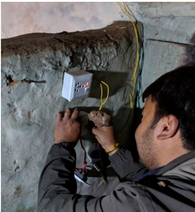
A technician upgrades kitchen electrical wiring for induction stove use.
