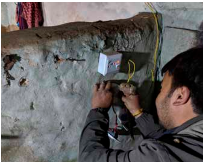
A technician upgrades kitchen electrical wiring for induction stove use.
